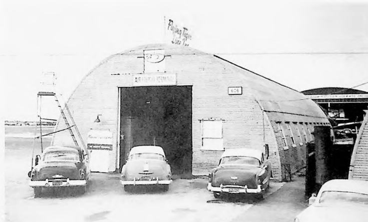
(B) The OAK station, located across San Francisco Bay from the SFO station, is housed in this quonset building at Oakland Municipal Airport.
