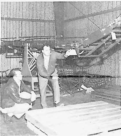
3. Arthur Harmison (right), cargo handler, and Agent Dick Spinney look over a new electric cargo conveyor, which does a fast job of loading or unloading freight directly between truck and aircraft on package freight and flowers. SFO is the system's largest source of flower traffic.
