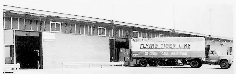
2. Here is a street view of FTL's air freight terminal at Philadelphia International Airport, with FTL trucks and a Yale & Towne truck, one of our largest shippers, lined up at the truck-bed high dock. FTL's facilities here are among the most modern in the nation. They are located in a block-long brick building, newly built for handling air express, air freight and mail. All carriers serving the airport have their freight facilities concentrated in this building and another adjoining it.
