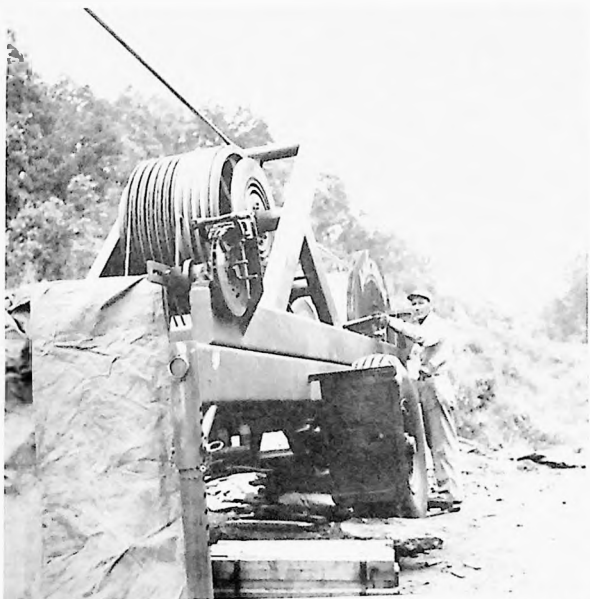
The stringer assembled and ready for action in the field.
