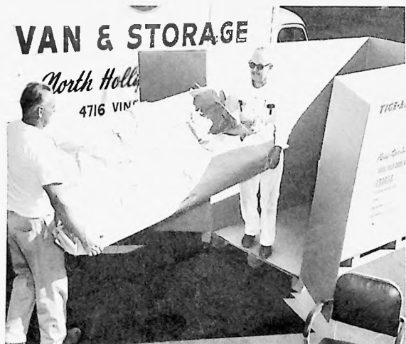
Container opens at top and end for easy stowing of household goods.
