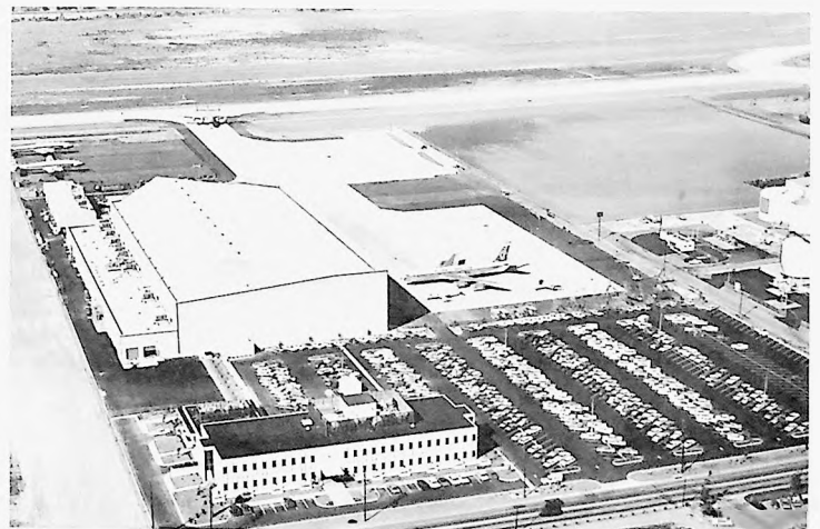
AFTER. An aerial view of FTL's new world headquarters in Los Angeles shows the modern office building in the foreground and the mammoth hangar and equipment buildings in the rear. On the ramp is a Boeing 707 jet capable of more lift than the original fleet combined
