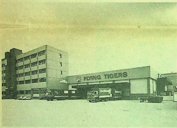
Exterior of Flying Tigers' new terminal and office complex in Frankfurt, West Germany, above.
